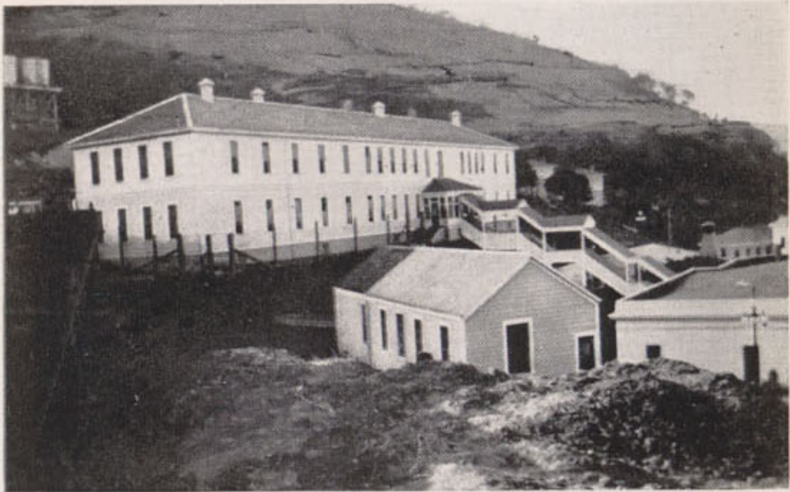
The Chinese Detention Building at Angel Island.
