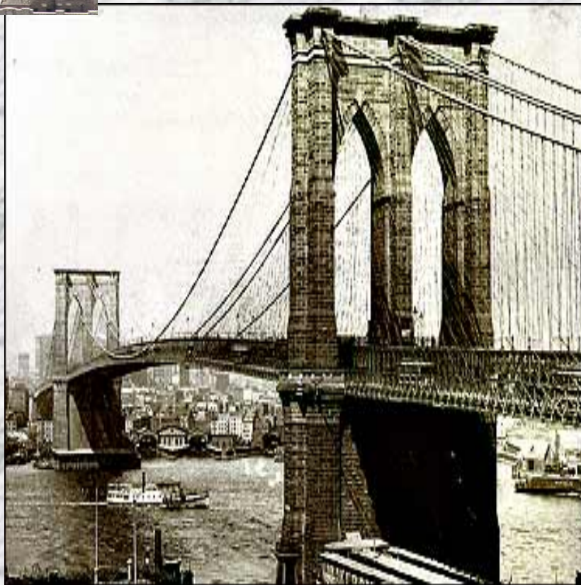
BROOKLYN BRIDGE SPANS 1595 FEET IN NYC
